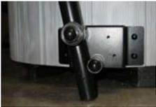
**Note:** Brackets must be mounted horizontally, with the angle mounted on the radius of the spa.
