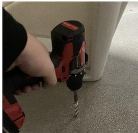
6. Clear all anchor holes of any debris. Shop-vac may be required if debris gets in anchor holes.
