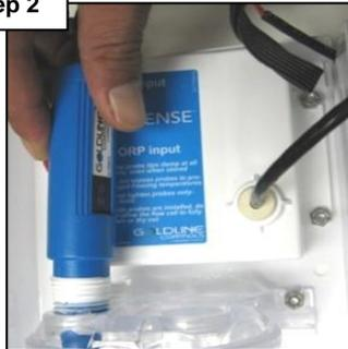
Unscrew & remove the probes from the flow cell chamber.
