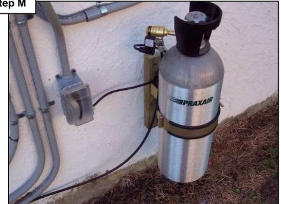
If the valve continues to release CO<sub>2</sub> despite the absence of power replace the valve (AQL-CHEM2 or AQL-CHEM2-240).
