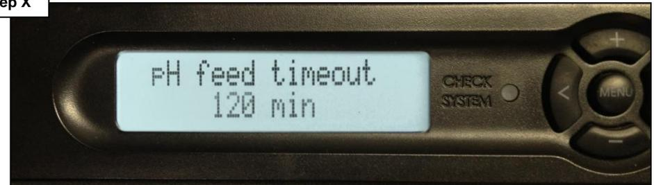
Go to 'Chemistry Config. Wizard' press plus button to enter, scroll to right until 'pH feed timeout' option appears. Press the (+) button to extend up to 120 minutes. Once complete, follow instructions on page 7 to reset the 'Timeout Error'.
