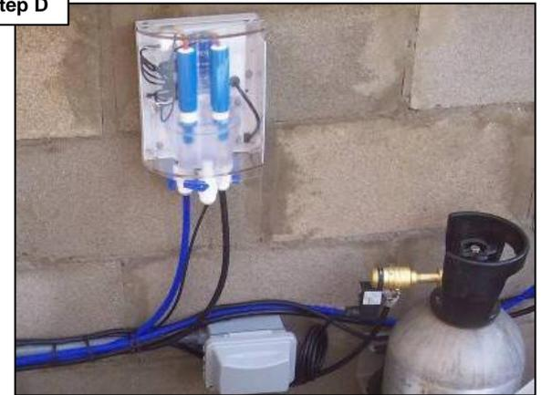
If the flow cell is in direct sunlight, relocate it or reduce sun exposure (extreme heat can cause a 'CSM Comm Error'). If this does not correct the problem or it is not in direct sunlight, replace the module (GLX-SD-ELEC-MOD).
