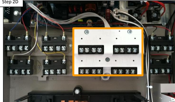
**When installed in an OmniLogic, lights should either all be ON or all OFF the relay bank. IF light are wired into mixed relays, correct and retest. IF not mixed, & resyncing does not correct, replace out-of-sync lights.**
