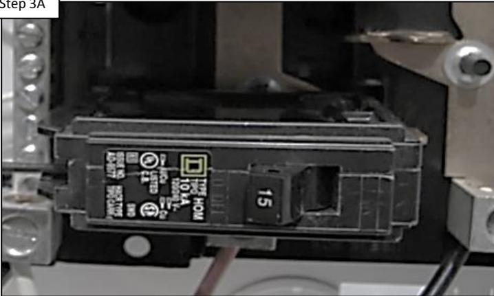
Power the lights down for a minimum of 2 minutes either through the breaker or through the controller. After restoring power and cycling, IF lights are still dim/flashing, go to step 3B.
