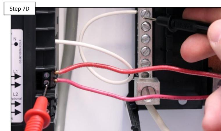
Test the module for 120VAC by checking either terminal to neutral. IF 120VAC is present, power cycle and replace the module if the problem persists (AQL-COLOR-MODHV). IF not, correct source power issue.
