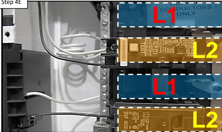
The source power that is provided to the lights needs to be on the same bus as the power provided to the module. Verify they are. IF power is not on the same bus, correct and retest. IF correct, go to 4F.
