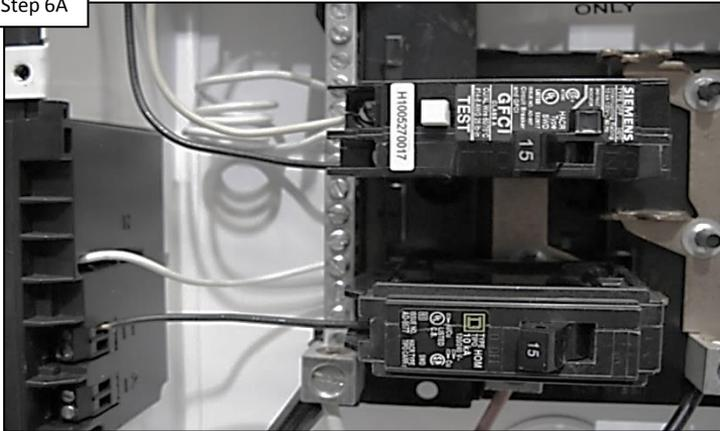
Power the lights down for a minimum of 2 minutes either through the breaker or through the controller. After restoring power and cycling, IF lights are still dim/flashing, go to step 6B.
